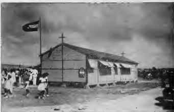
Army bombhouses have been used for many things besides sleeping quarters. The one shown here is now a place of worship for the San Nicolas congregation of the Anglican Church. The addition of an attractive altar, some pews and a tiny organ makes an acceptable church until construction can be started on a new one.
